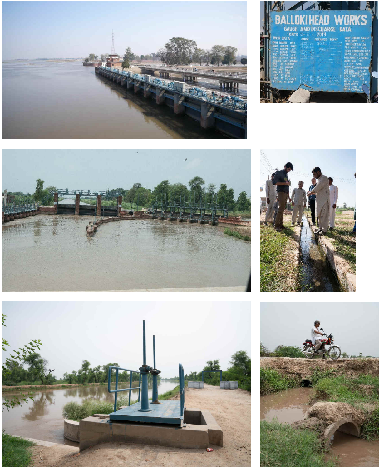
Figure 4.2: Hierarchy of canals in the study area canals from head works, mains, branches, distributaries to watercourses for field application. © FiW
