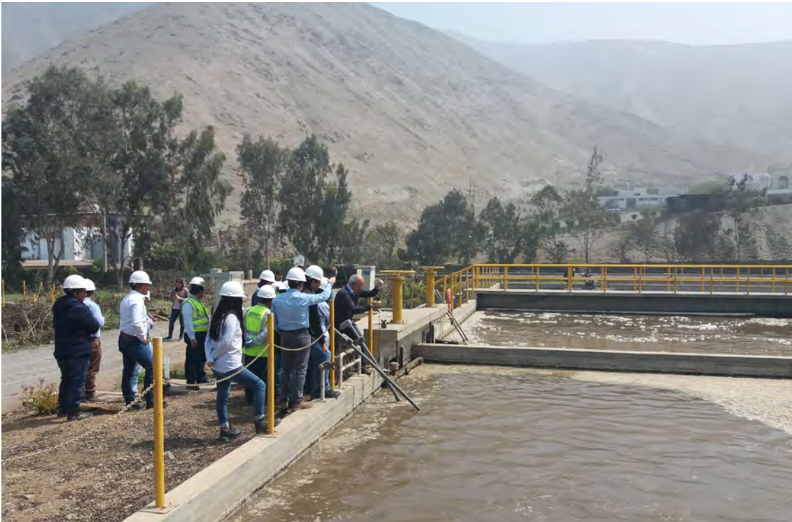
» Figure 6.3: Field visit to the wastewater treatment plant Cieneguilla. Picture: C. D. León.
