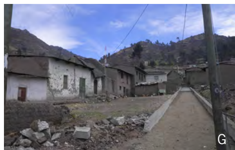
» Figure 4.6: Hazard analysis of the springs in Tupicocha, October 2019. (A) Map showing the springs, the land use and the places of the pictures, (B) Spring 1 Chiribamba, (C) waste near spring 1, (D) spilled oil, (E) tank with unknown liquid, (F, G) livestock (Pictures: M. Krauss (B) T. Fischer (C-G)).
