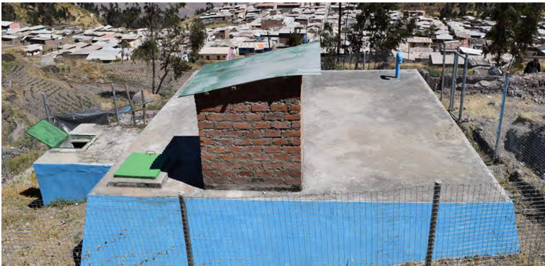
» Figure 4.4: Water storage tank of Tupicocha with a shed for chlorine dosage on top. Picture: M. Krauss.
