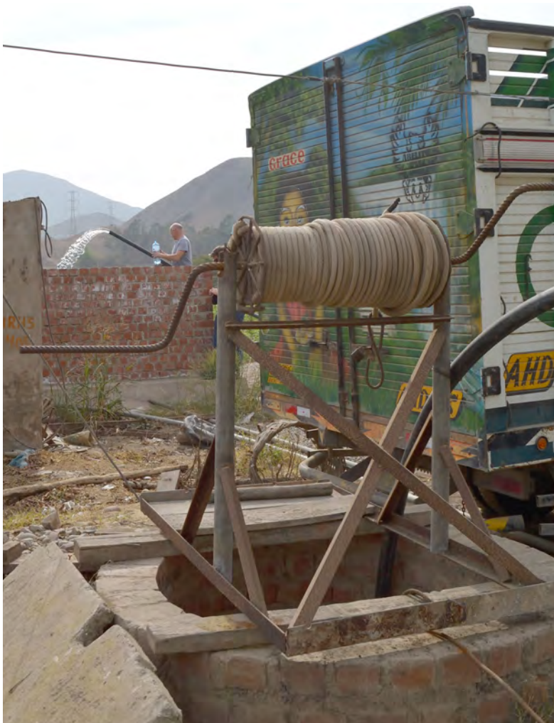
» Figure 5.5.: Open dug well in the lower Lurín valley (Manchay). Picture: M. Krauss.
