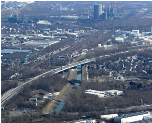
River Emscher in Bottrop: intensive land use on both sides of the river hampers renaturalization.
