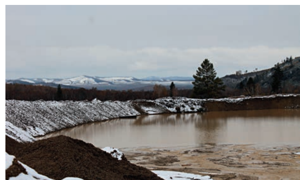
Catchment basin for unpurified wastewater from mining activities in the Kharaa River catchment in Mongolia
